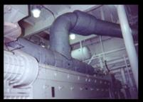
Manifold, Exhaust & Expansion Joint
