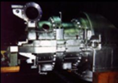
Elliott Compressor Before
